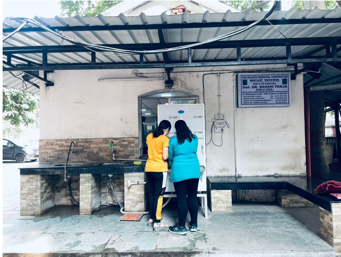
Installation of water dispensers in the college premises donated by the Hon'ble MIC, Dr. Shashi Panja
